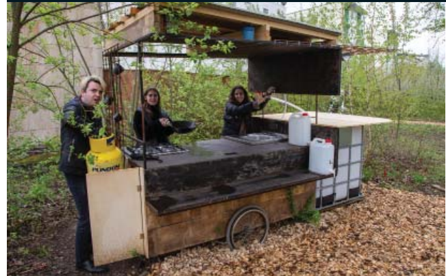
Figure 3 and 4: From conceptualization and planning to implementation: the workshop on reuse and circular design took place in the construction pit »Krater« in Bežigrad.
