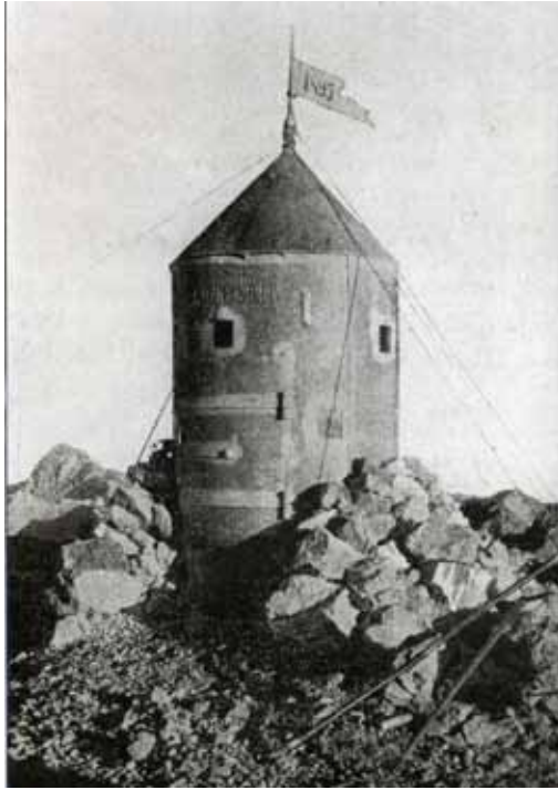
Figure 6: In 1895, Jakob Aljaž, the parish priest in Dovje, bought the summit of Triglav (16m2) for one gulden and erected a tin tower that was less than two meters high and one meter wide. It had two main functions: serve as a shelter that could accommodate a few mountaineers in the event of bad weather; and serve as the highest Slovenian blaze during the battle for the mountains between the Slovenes and Germans. Photo archive: Slovenian Alpine Museum in Mojstrana.
