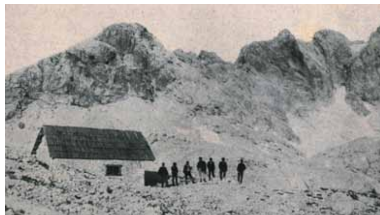
Figure 1: Shelter on Prodi (near the present-day Planika hut) was known as the 'Triglav Temple' due to its astonishing views. It was built in one month by Jože Škantar-Šest and his son Lovrenc in 1871 on the initiative of enthusiasts from the clique of 'Friends of Triglav'. The small stone building was built at an altitude of 2,404 meters, surfaced with sand on the outside and covered with shingles. There was a bunk bed for six people and a small open fireplace. On September 18, 1871, it was ceremoniously opened by a handful of mountaineers. Photo archive: Peter Mikša.
